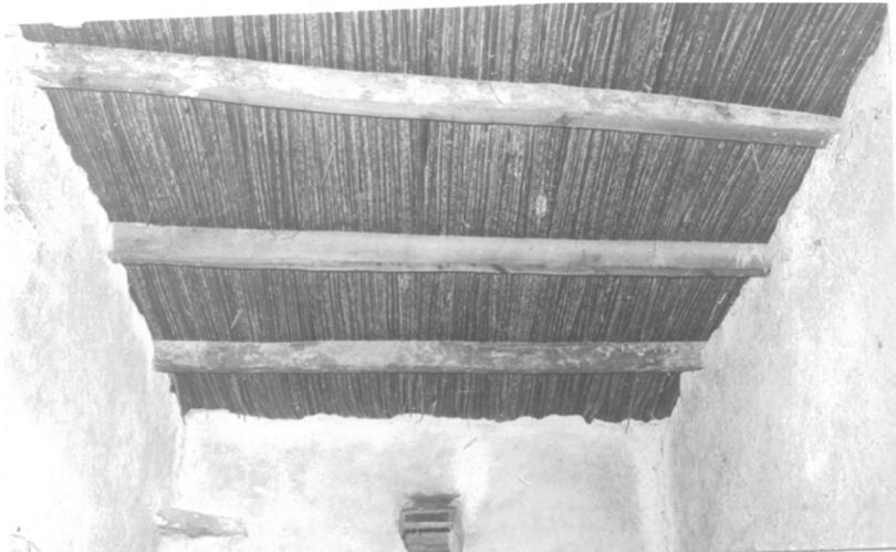
Fig. 2. A mat of palm midribs in the roof of an Araishi house [8].
